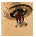
When the air temperature above the fire rises to a certain temperature, a fire sprinkler system is activated. The sprinkler sprays water forcefully over the flames, extinguishing them completely in most cases, or at least controlling the heat and limiting the toxic smoke until the fire department arrives. Only the sprinkler(s) nearest the fire activate. Smoke alone does not activate sprinklers.
